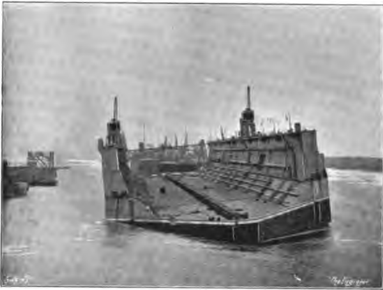
Fig. 512.—Dock Heeled to remove Starboard Connection.
